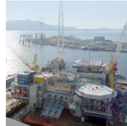
Gjea topside at Stord, Norway.
