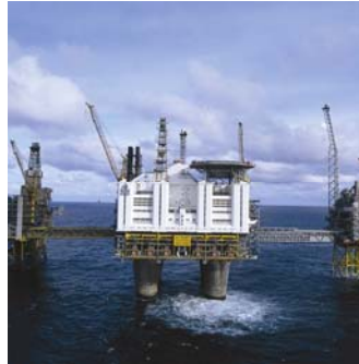
StatoilHydro awarded Aker Solutions an engineering, procurement, construction and installation (EPCI) contract for upgrading the drilling facilities on the Oseberg B platform in March
