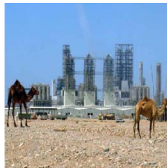
Yansab world scale polyolefins project: First Western/Chinese JV project in Saudi Arabia; in Q1 the first Polypropylene pellets were produced and the product handling unit was completed
