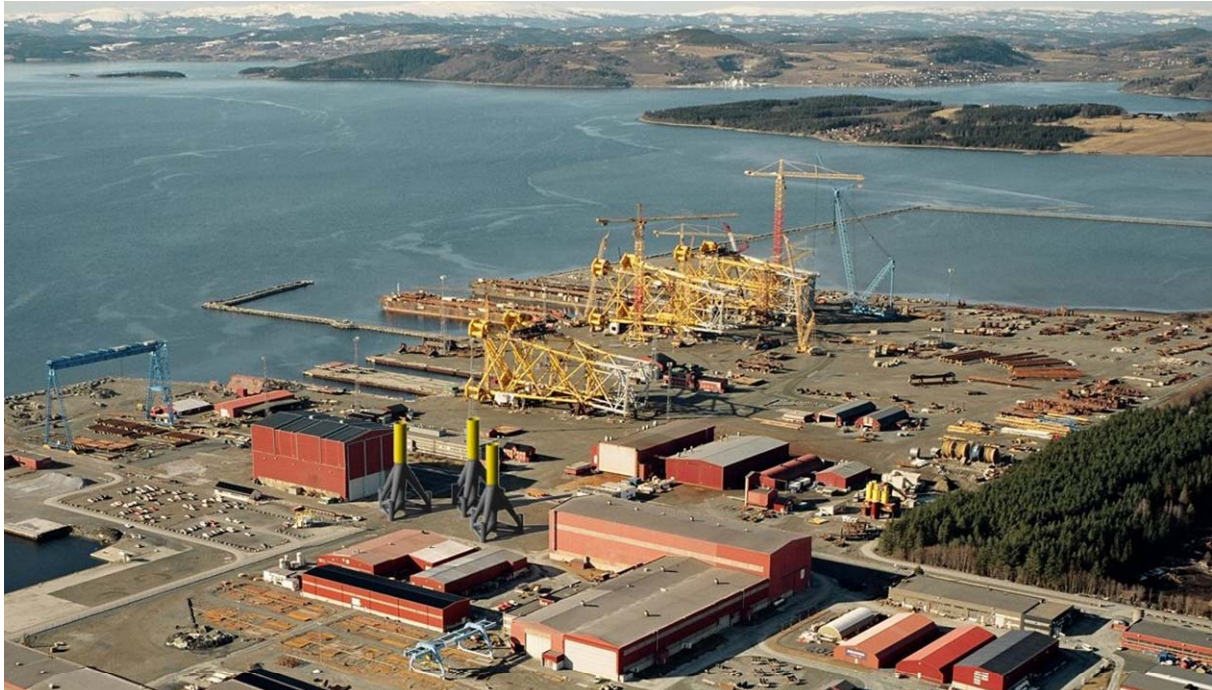
Three substructures are included in the picture above from spring 2005 showing the three Buzzard jackets in order to illustrate the size of the substructures for the offshore windmills.
