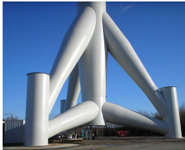
The picture above to the left shows two Multibrid M5000 (5MW each) windmills in Bremerhafen, these windmills are prototypes for the complete offshore windmill including the substructure. The picture above to the right shows a close-up of the substructure.
