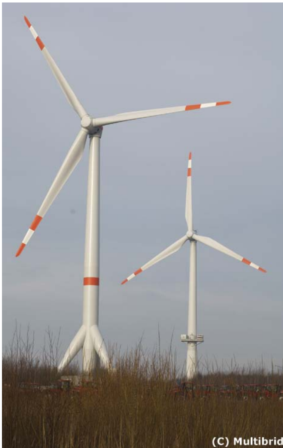
The picture above to the left shows two Multibrid M5000 (5MW each) windmills in Bremerhafen, these windmills are prototypes for the complete offshore windmill including the substructure. The picture above to the right shows a close-up of the substructure.
