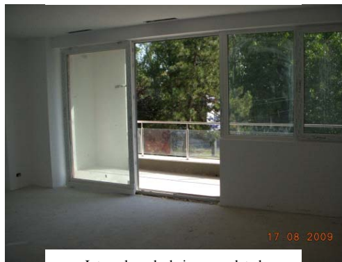
Internal works being completed
