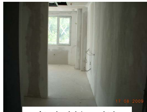
Internal works being completed
