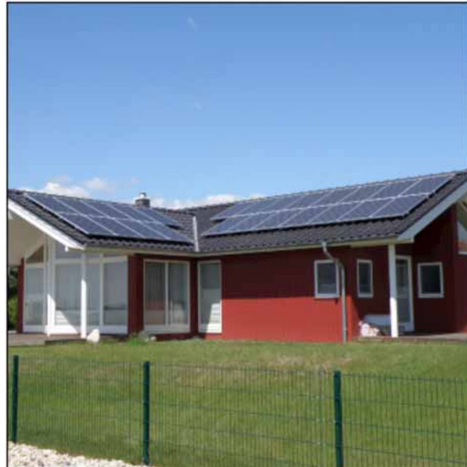
Photo: A Sovello installation in Mühlbeck, Germany
